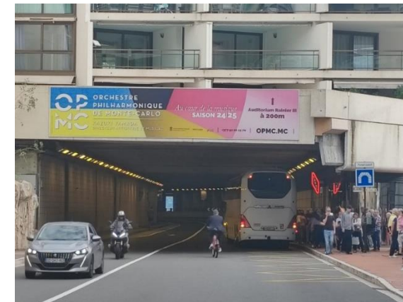
Footbridge banner Tunnel Louis II
