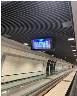
12 screens along travelateurs LCD screens 32"
